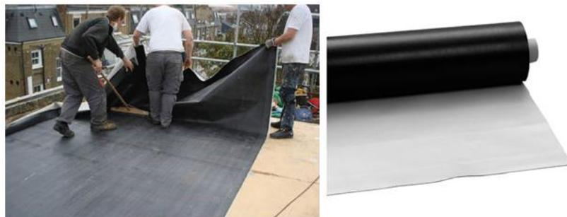
**Photo11. Polymer waterproof membrane arrangement on the synthetic base**
