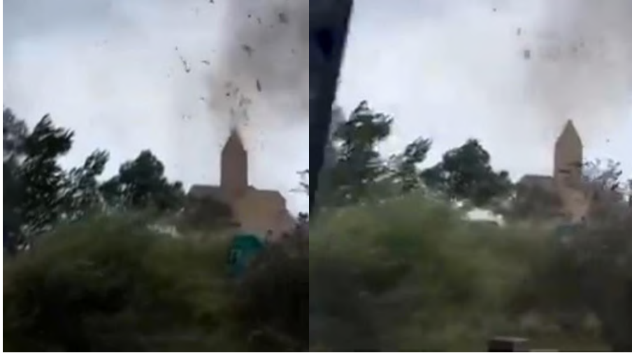
Fig. 5. Removal of the covering of the dome of the Alaverdi Cathedral. The time interval between frames is 1 second. Video source: https://www.youtube.com/watch?v=ZFvYlzEhBr4 .
